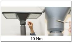
2. Prepare the luminaire for the instalation.
