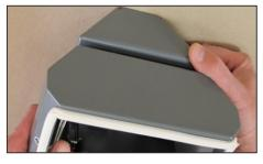
9. Screw the luminaire cover back on. To maintain the correct sealing function, make sure that the screws are tightened evenly.
