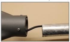
10. Take out an inner adepter from the bottom part of the luminaire. Fix the luminaire on the post. Tighten allen screws with tightening torque of 8 Nm.
